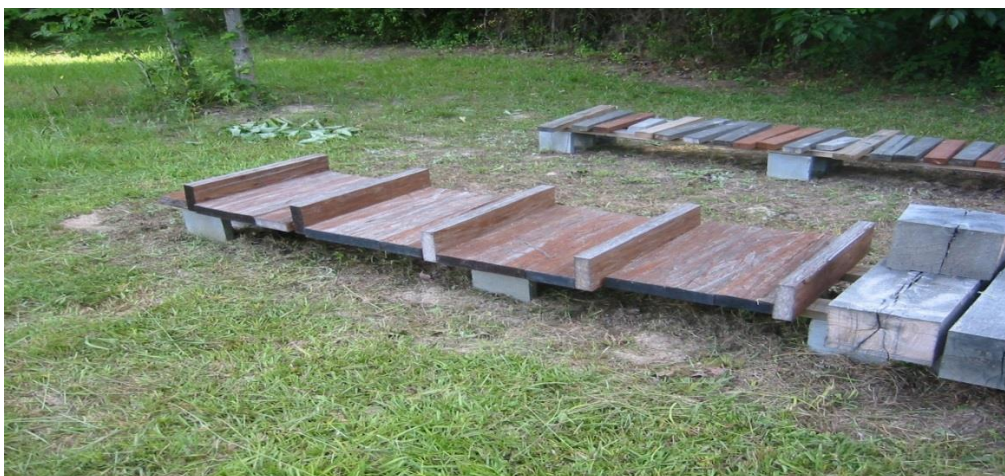
Fig. 7. Samples of SPSL, treated with silane-based WRP, after five years of aboveground exposure in AWWA Hazard Zone 4
