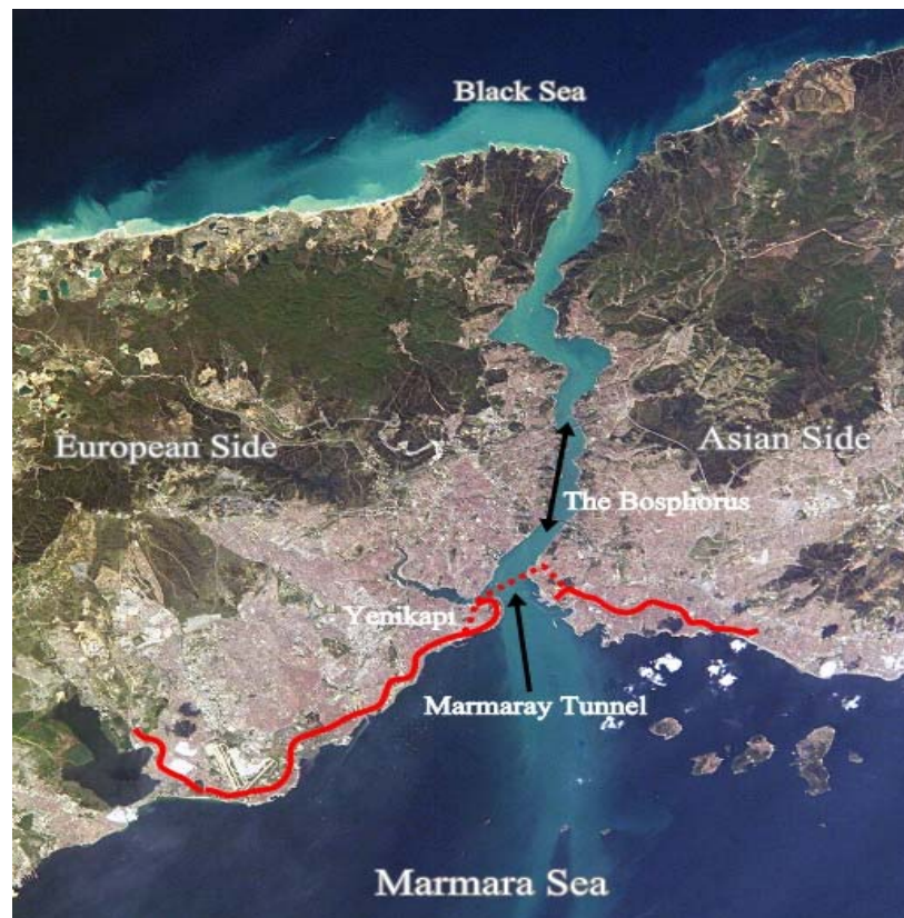
Fig. 1. The Marmaray Project along the coast line of the Marmara Sea and Yenikapi excavation area
