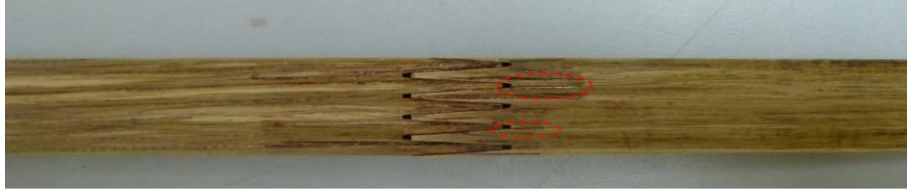
Fig. 7. Bending failure mode of finger-jointed BLVL. Failure zones are outlined with dashed red ovals.
