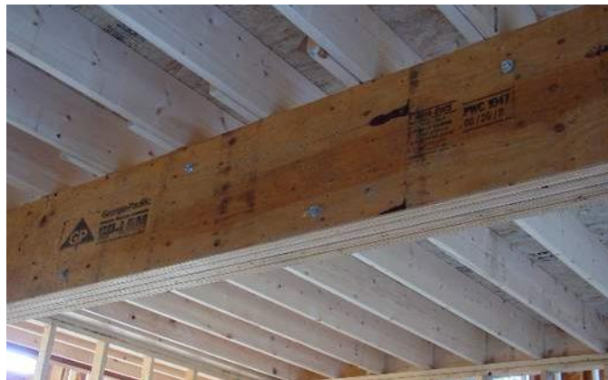
Fig. 1. Use of LVL beam in a structure
