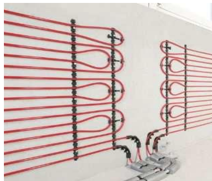
Fig. 2. Installation of a wet system (Rehau, 2013a)
