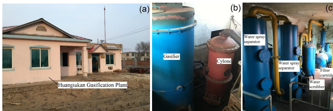
Fig. 1. Pictures of the gasification plant (a), the downdraft gasifier (b) and the scheme of the layout of this plant (c)
