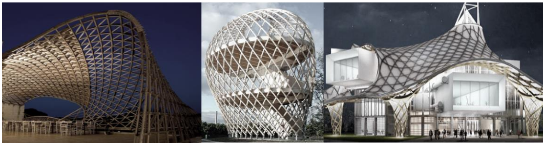
Fig. 1. Left picture is the Toledo gridshell (Gridshell.it 2012), middle picture is the Helsinki Zoo's observatory tower (Paoli 2007), and right picture is the Centre Pompidou Metz (Lewis 2011).
