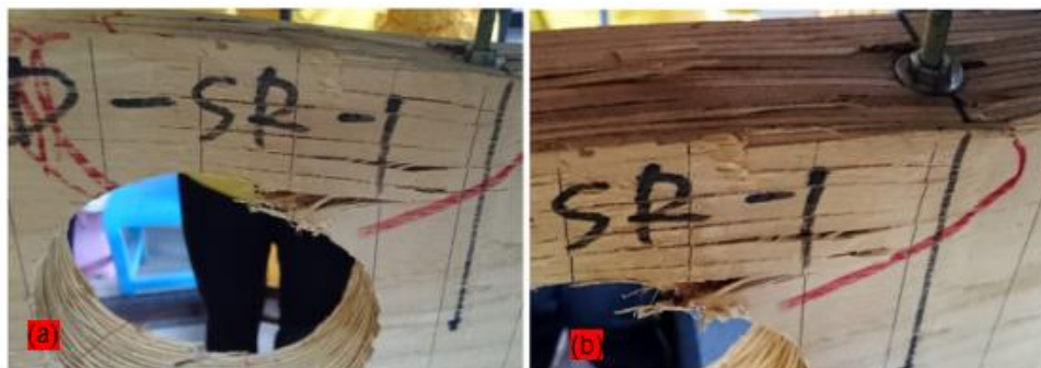
Fig. 11. Cracks above the hole were confined within the two rods (a), and the wood under the washer was compressed (b)
