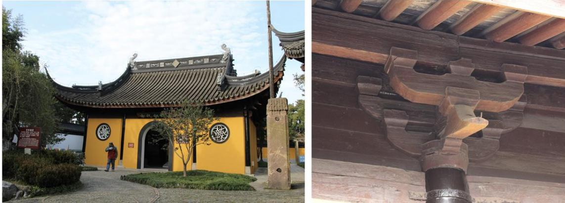
**Fig. 1.** Tianwang Hall and its typical Dou-gong bracket on top of the column
