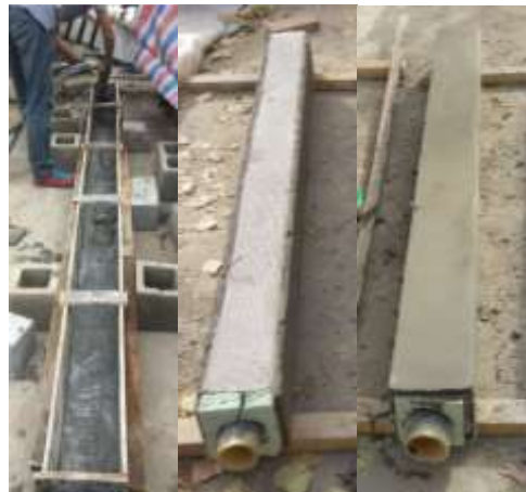
Fig. 11. Manufacturing process of the composite beams
