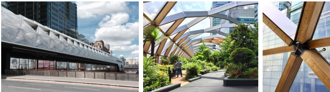
Fig. 2. Crossrail Place, Canary Wharf, London, UK
