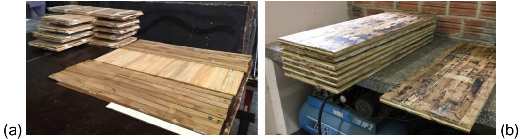
Fig. 3. Panel production: (a) gluing of strips, and (b) finished cross-laminated timber-bamboo
