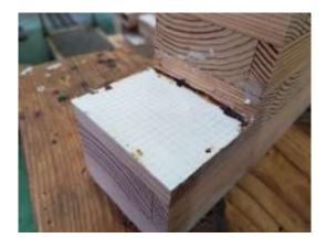
Fig. 6. Half-lapped connection reinforced with GFRP
