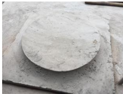
Fig. 3. Plinth ruins in the renovation of Nanjing Drum Tower (Nanjing, Jiangsu, China).
