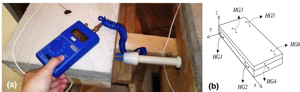
Fig. 5. (a) Measurement of the timber moisture content; and (b) position of the measuring points
