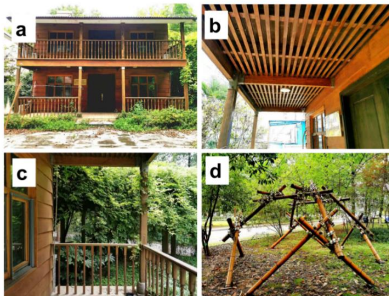
Fig. 5. Bamboo use in buildings and structural construction: a) bamboo building, b) bamboo ceiling, c) bamboo exterior, and a d) bamboo structure (Location: Nanjing, Jiangsu Province).
