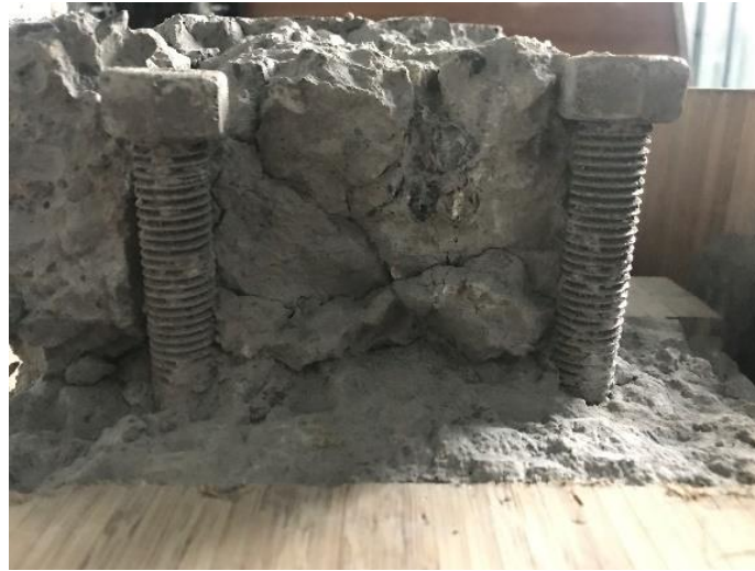
Fig. 6. Intact connection between screws and glubam
