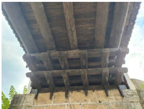
(c) Detail of cantilever system
