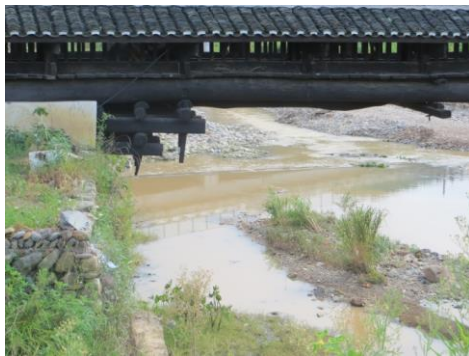
(a) Cantilever system on abutment
