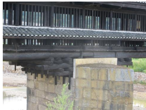
(b) Cantilever system on pier
