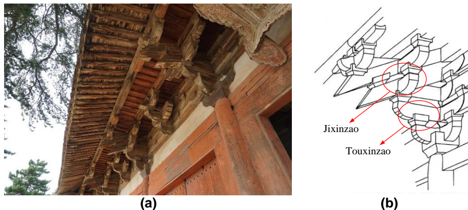
Fig. 3. The Dou-Gong bracket at column top in the East Hall of Foguang Temple: (a) exterior photo; (b) the structural form of Jixinzao and Touxinzao Dou-Gong bracket
