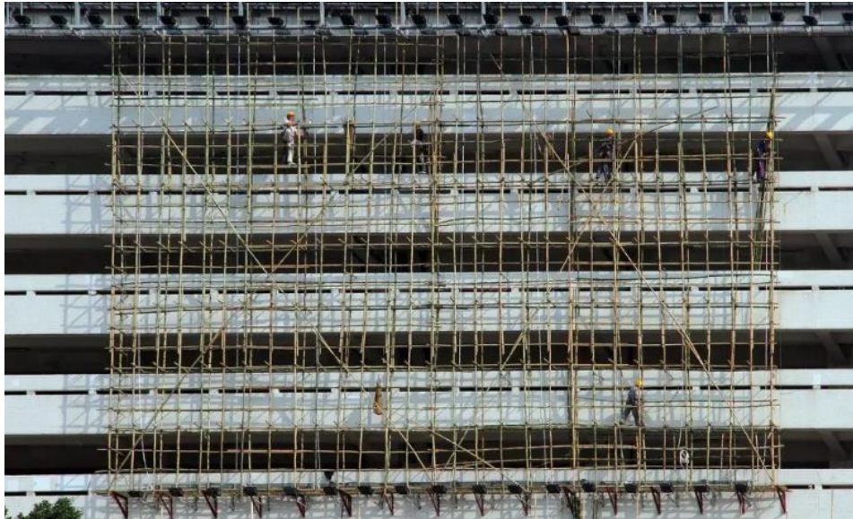
Fig. 2. Bamboo scaffolding (Neumann 2020)
